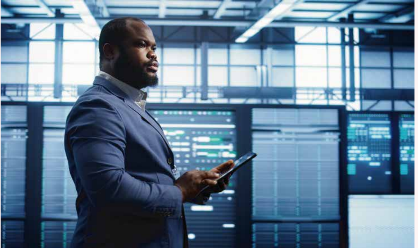
A technician walking in server room doing checkup inputting data
